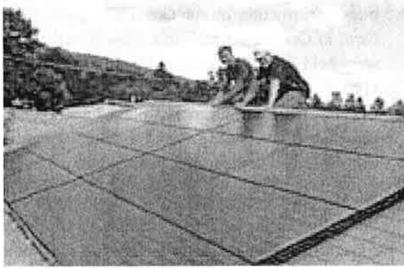
Solar panel installation, Cabot School, Cabot, Vermont.
